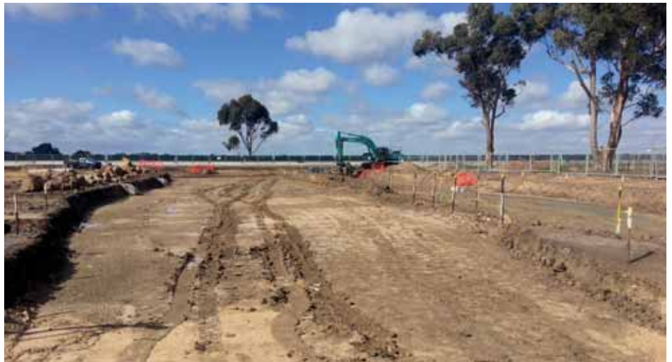
Construction of St. Georges Boulevard - Merrifield Living
